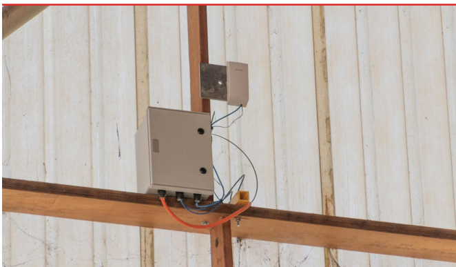
Picture 3: Wireless Access Points at both ends circled in RED. Closest WAP in picture is at control room end receiving signals of 2 cameras. Line of sight distance approximately 200m.
