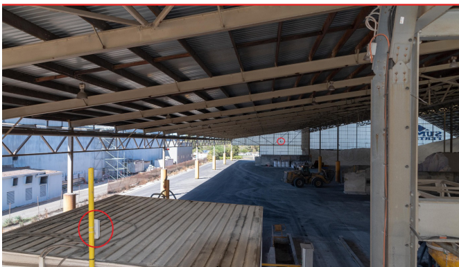
Picture 3: Wireless Access Points at both ends circled in RED. Closest WAP in picture is at control room end receiving signals of 2 cameras. Line of sight distance approximately 200m.
